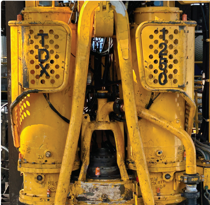
The West Auriga's mainwell TDX-1250 equipped with Nanoprecise IoT vibration sensors.
